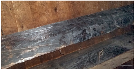
An opening in the basement's modern drop ceiling reveals charred beams salvaged from the burned church and incorporated into its successor.
